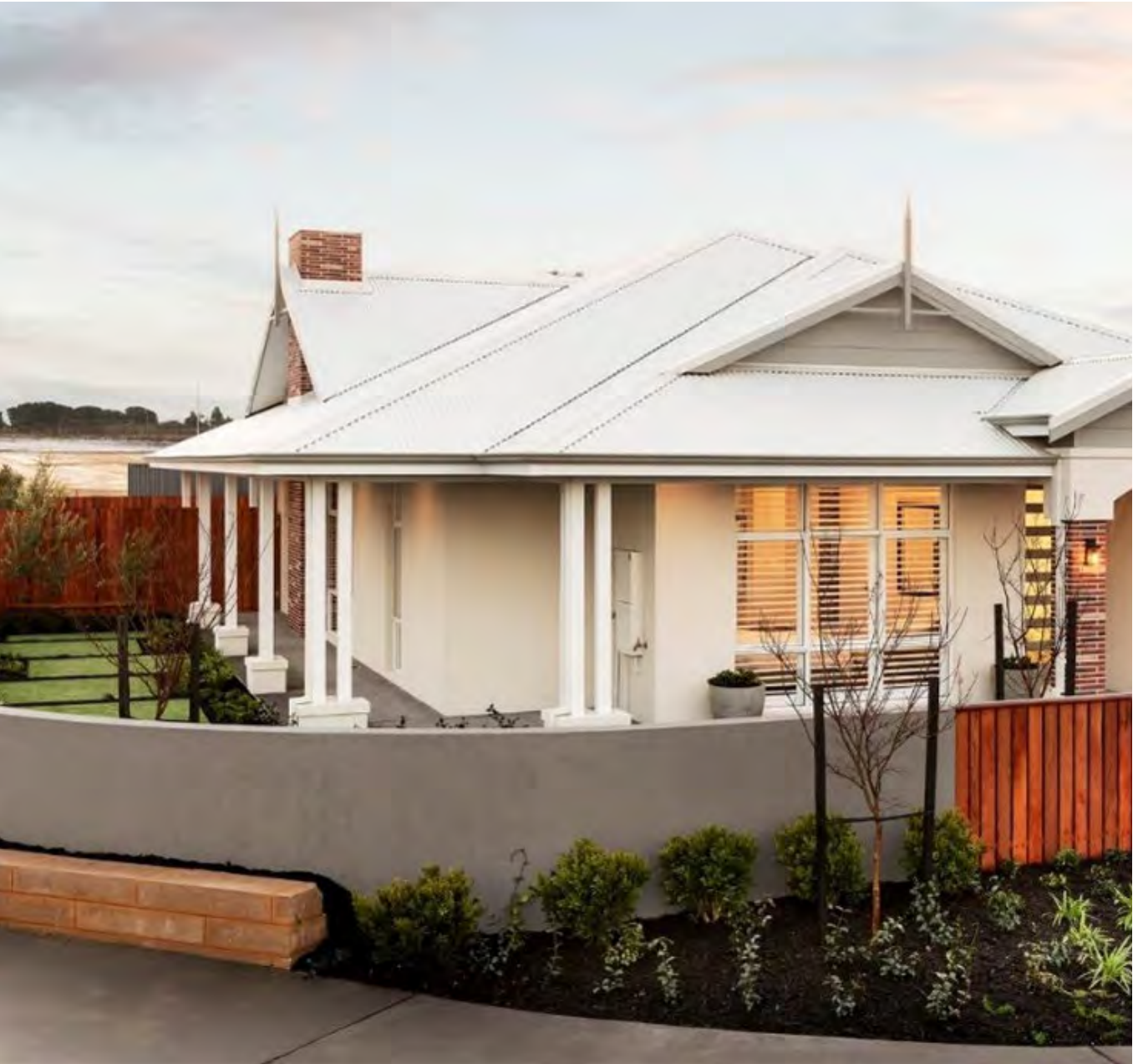
Extending a verandah along the secondary elevation improves the visual presentation of a dwelling at a street corner.
