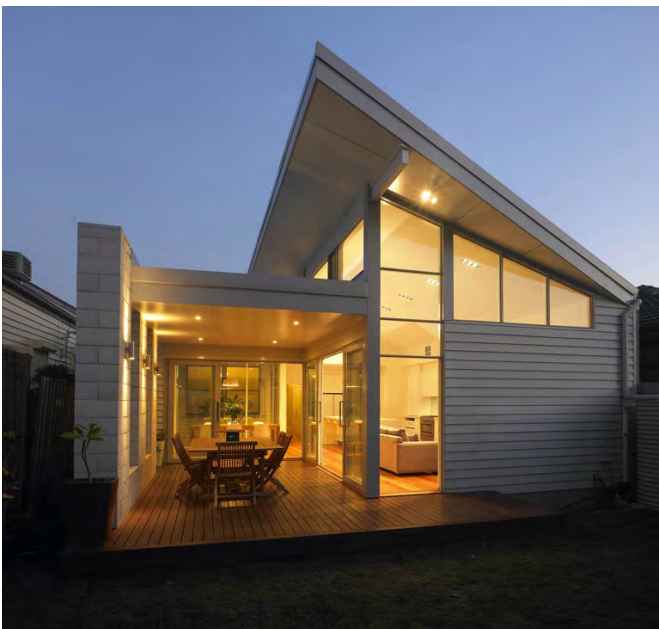
Skillion roof and extended north facing windows improve passive heating during cooler months.
